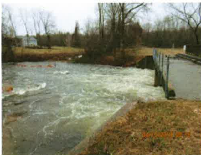
Photo 55 Downstream View of Bennett Dam
